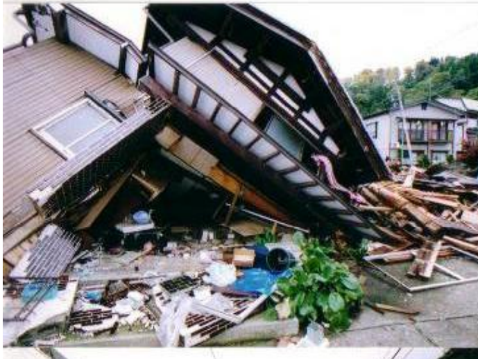
The Area Damaged by the Chuetsu Earthquake in October 2004
