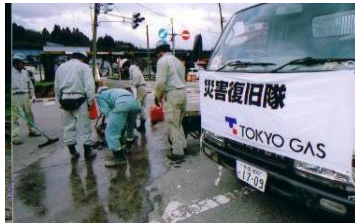
Gas Restoration Crew in Niigata, October - November 2005
