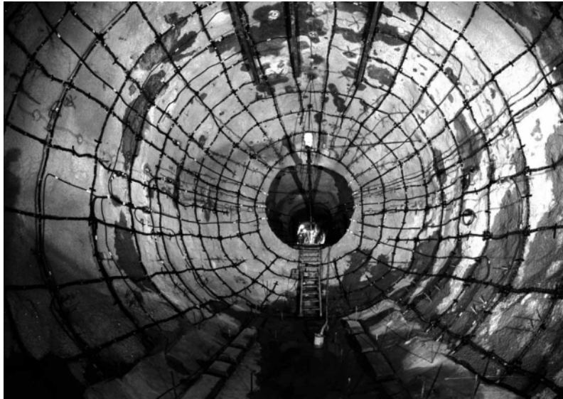
Photo 1: Excavated test cavern
