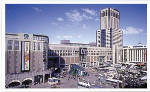
Regional air-conditioning systems
