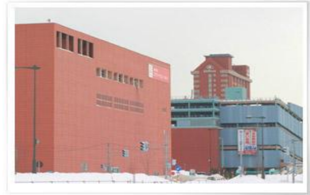
High-efficiency gas turbine power generation
